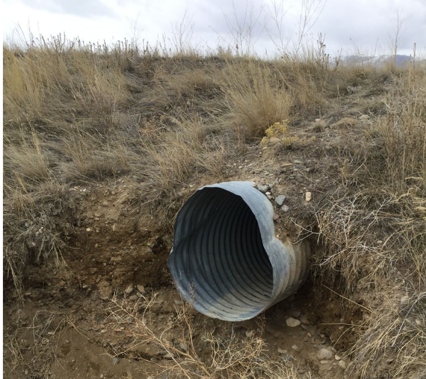
Photo 63: Corroded CMP culvert
