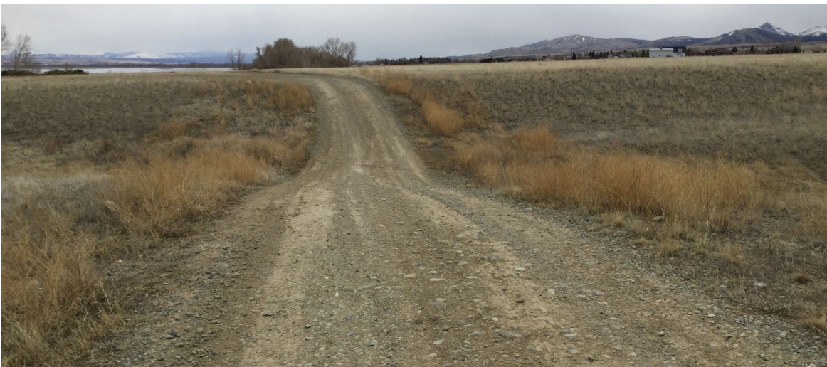
Photo 64: Large drainage swale crossing access road; no culverts in this location
